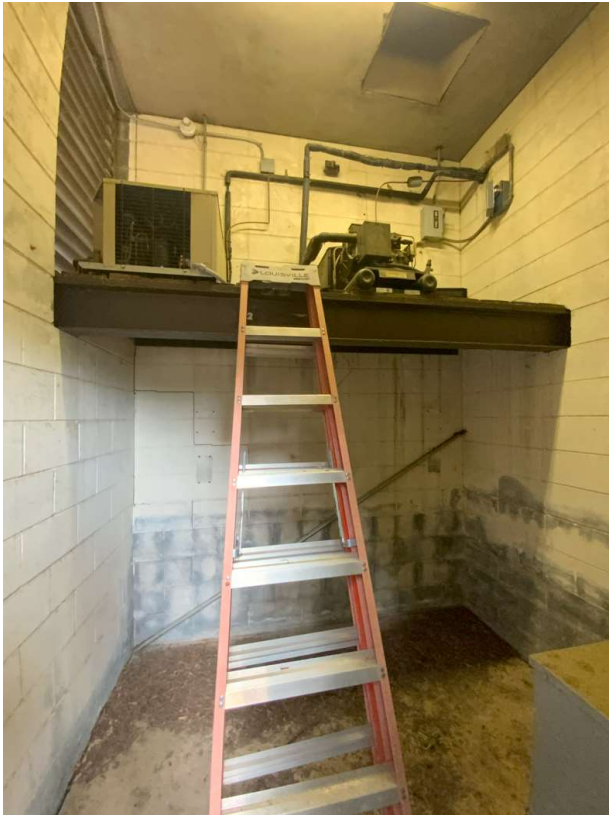
Existing compressors at Sherwood Elementary to be removed as Base Bid scope.
